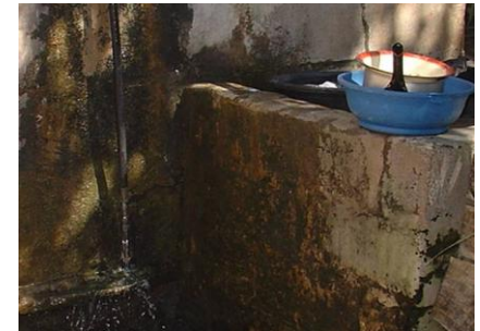
(Source: Courtesy KWSC Ltd.)
