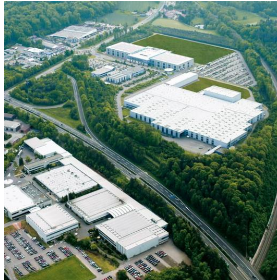
Festo Cylinderproduction and Customer Service Center, St. Ingbert
